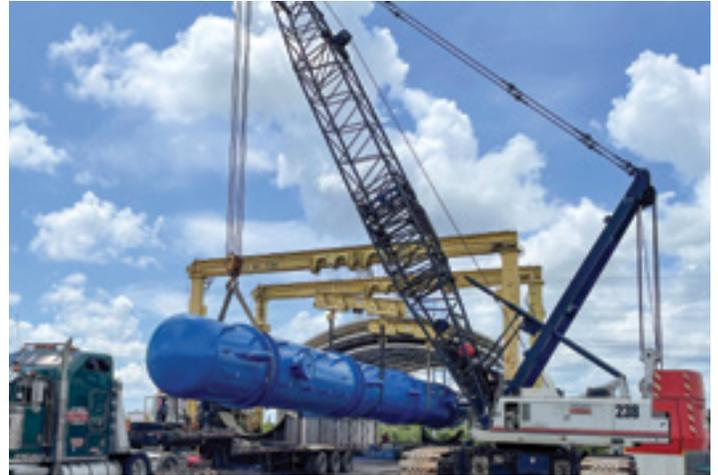
This bullet tank has complete joint penetration welds at all pressure connections, and our team performed well in ensuring top quality work for our customer.
