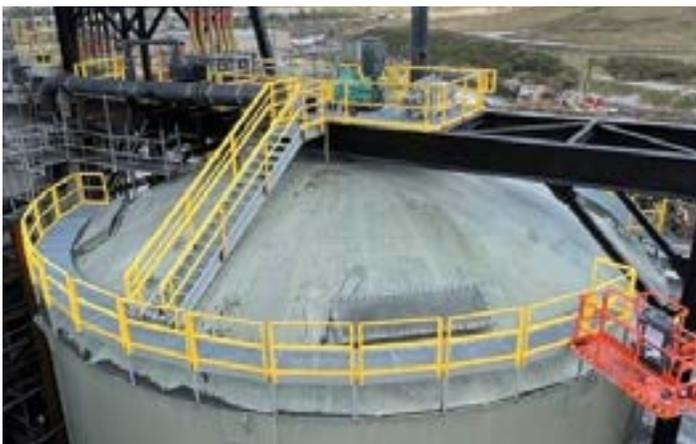
PB fabricated a 60' diameter by 32' high tank for a fertilizer facility in Mulberry, Florida. The tank consists of a flat bottom, a shell, and an umbrella dome roof design for two INWC vacuums, which were erected by the U.S. crew.
